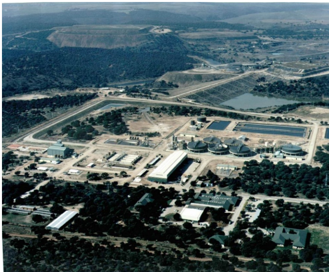
The old Quercus uranium concentrate manufacturing plant at Saelices el Chico.
