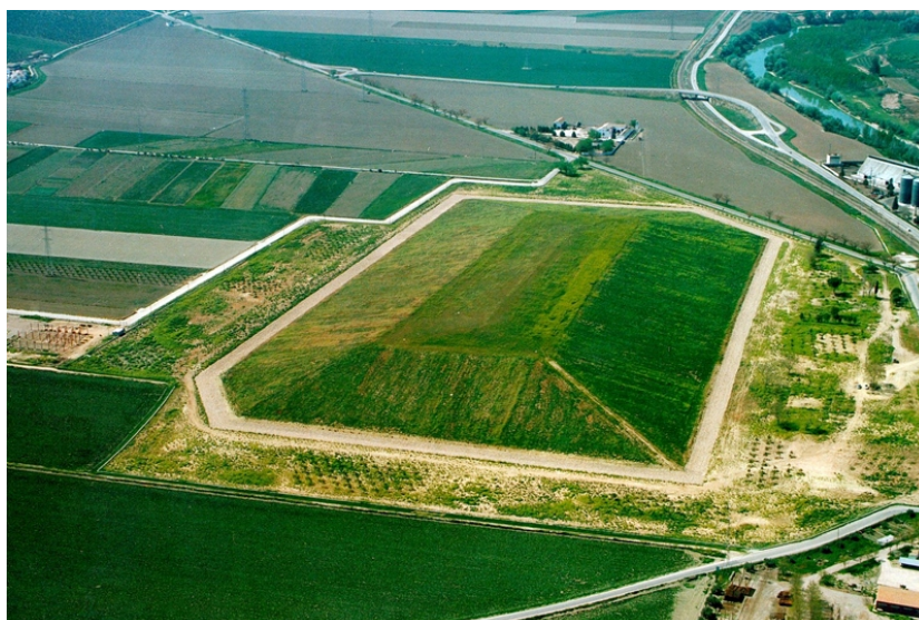
The restored site of the old Andújar uranium mill.
