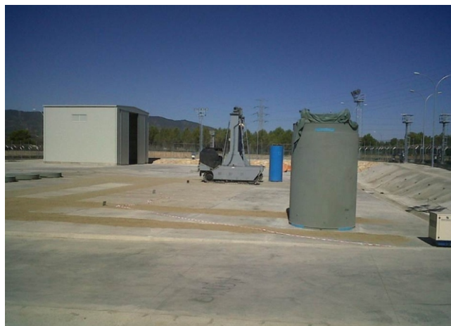
Ascó Nuclear Power Plant ITS facility.
